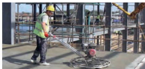
Figure 14. Power trowelling for a hard wearing finish.
