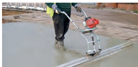
Figure 13. Petrol powered single beam screed
